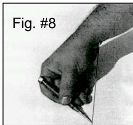
The most common probing method is to run a pointed, metal, hand tool along the edge of the seam with pressure to the tool. Some installers prefer to check seams with a compressed air tool which identifies a seam gap where air enters the seam and flutters the underside of the membrane.
